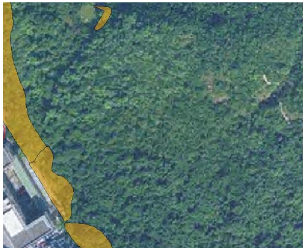
Figure 14 – Aerial photograph taken above a displaced landmass in hillside
