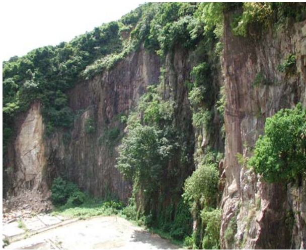
Figure 8 – Topographic survey of a rock slope with difficult access
