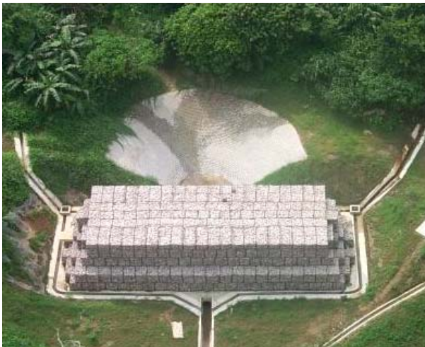
Figure 10 – Gabion debris barrier
