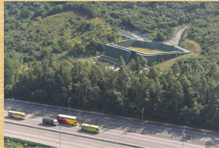
Building infrastructure to reduce urban flood risk during heavy rain events
