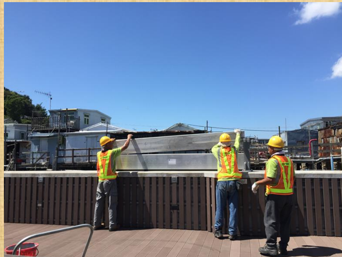
Installing flood barrier to cope with storm surges
