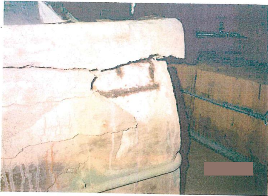
Concrete plinth before repair
