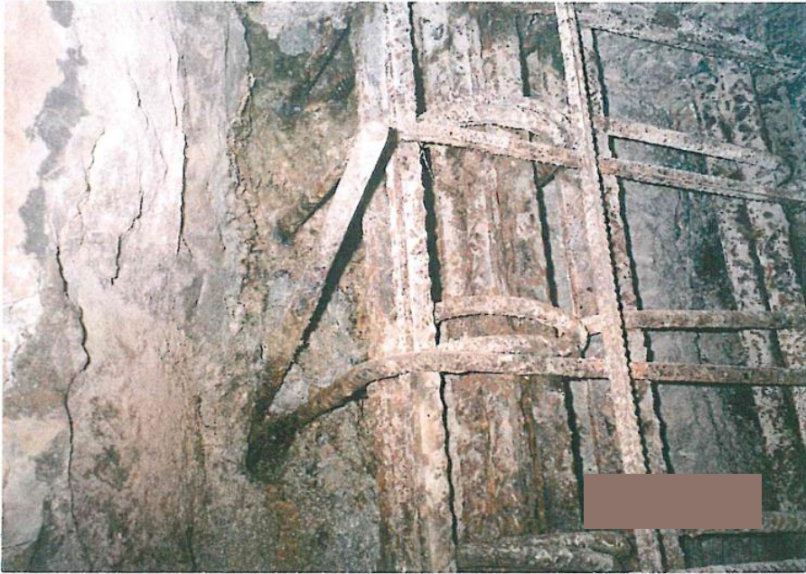
1200mm thick diaphragm wall condition after removal of the spalled concrete
