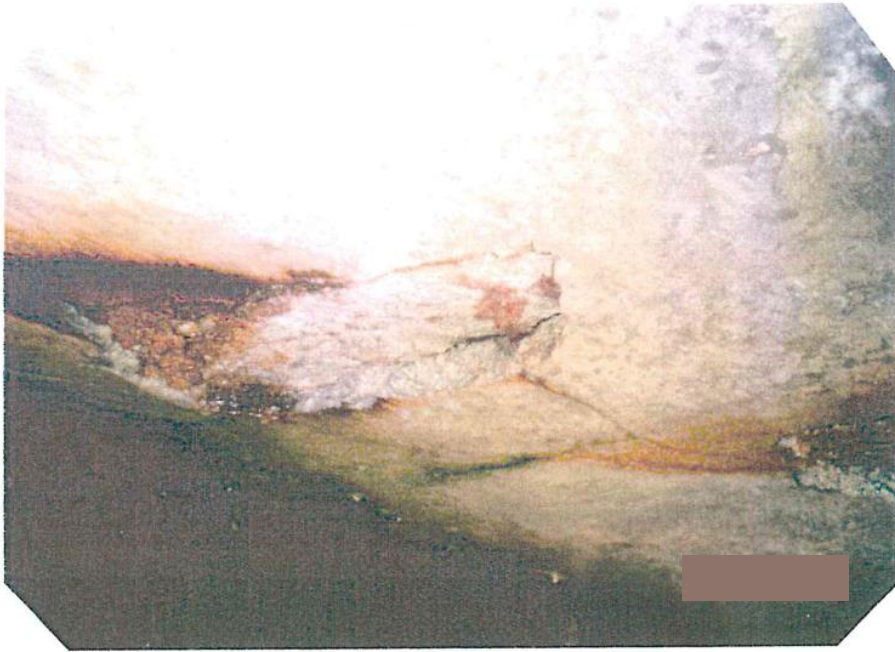
Concrete attack by sea water
