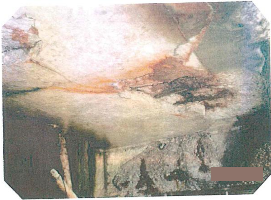
Concrete attack by sea water
