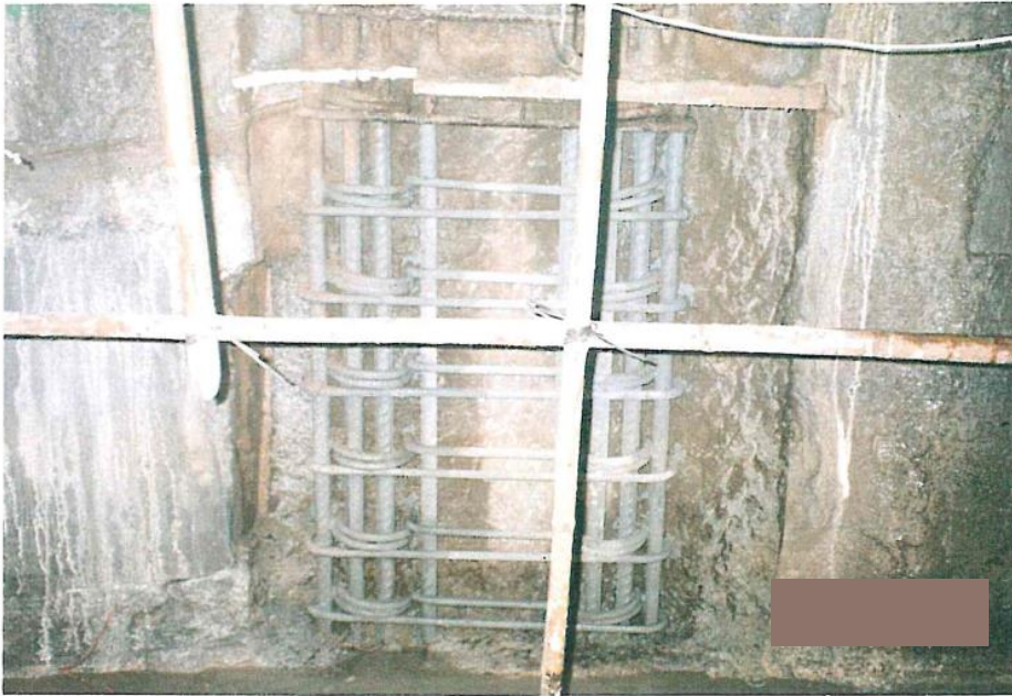
Steel bar primed after grit blasting
