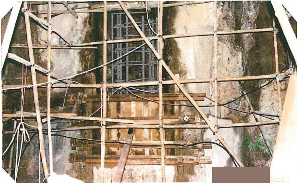
Formwork for recasting
