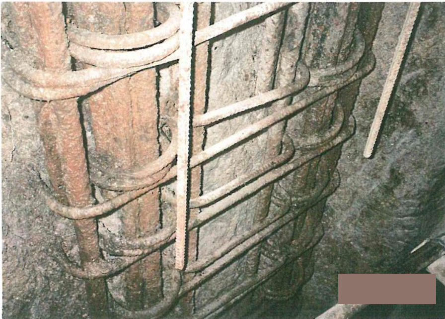
Steel bar condition after removal of the spalled concrete
