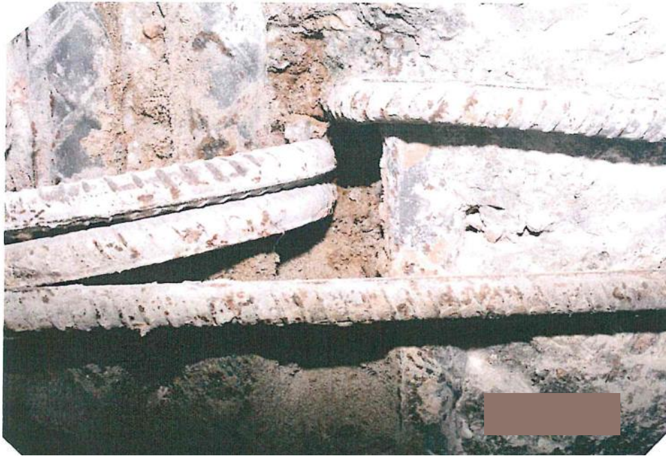
Deleterious/ muddy material within diaphragm wall
