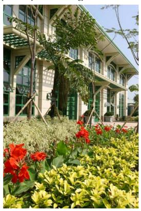
The design encouraged large roof overhangs and pergolas shading the facades bringing the OTTV values down to  $10.72 \text{ w/m}^2$  and  $12.64 \text{ w/m}^2$ . The structure of the appliance bay was selected as steel to allow visual integration of the design theme and the buildings services as well as economic benefits.
